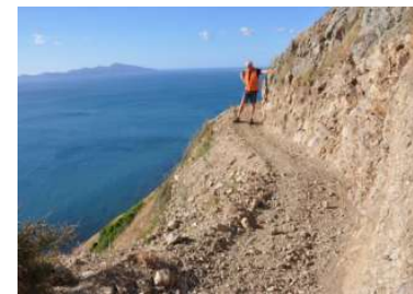
Constructing the track—Paul O'Hagan, Valley Landscape
