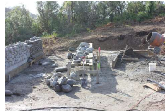
A beautiful rock wall under construction
