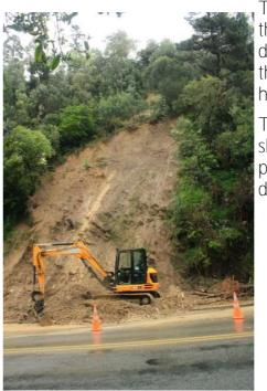
The slip scarp extended the full height of the hillside and covered half the road with debris. Luckily workers arrived shortly after the slip and, with rocks still sliding down the hill, cleared it.
